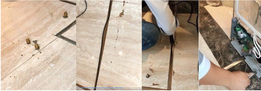
Install stainless scuff plate to fix the device.
